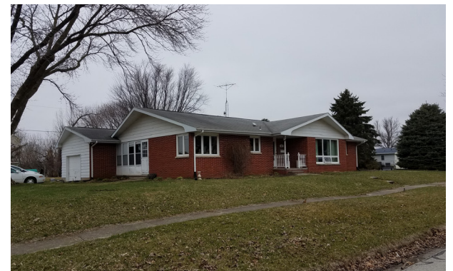
Repair and/or widen existing sidewalks where necessary
