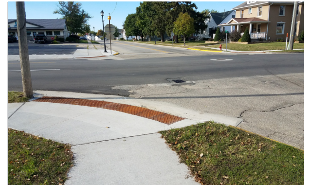
Continue handicap accessibility improvements
