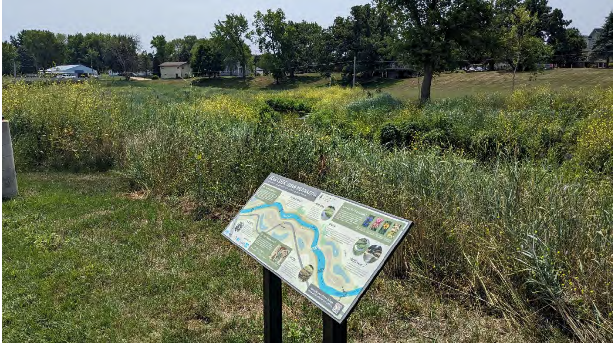
Photo point 15: Bear Creek restoration sign. Restored creek and riparian corridor in background. Date taken: July 11, 2023
