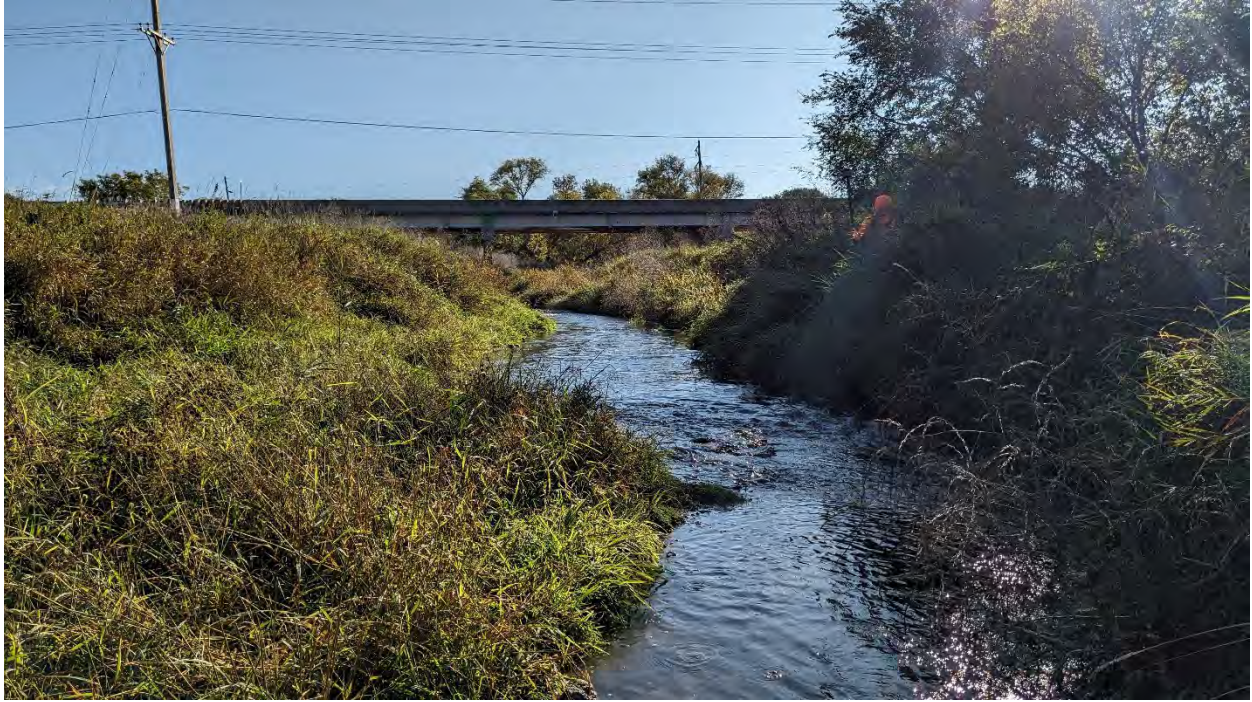
Photo point 3: Hewitt Creek facing east towards 11st St NE bridge. Date taken: October 10, 2023
