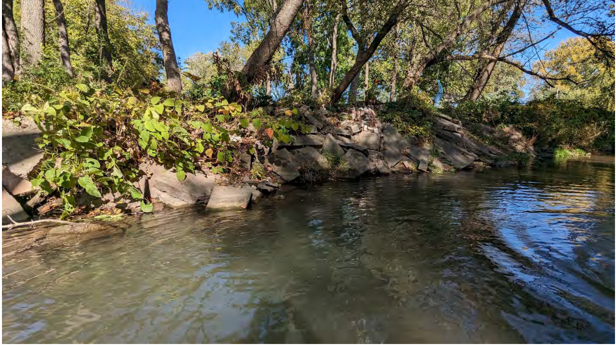
Photo point 18: Bear Creek looking south. Old pieces of concrete sidewalk used for bank stabilization. Date taken: October 10, 2023
